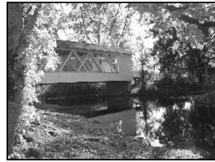
The Larwood Bridge
